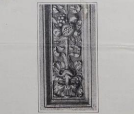
Fig. 5.—Metal-coated concrete molding.
