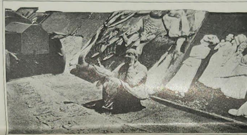
A clever bit of work done in sand and cement.
