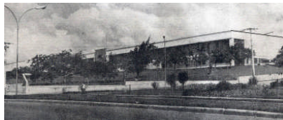
RCA plant on Avenida David Sarnoff
