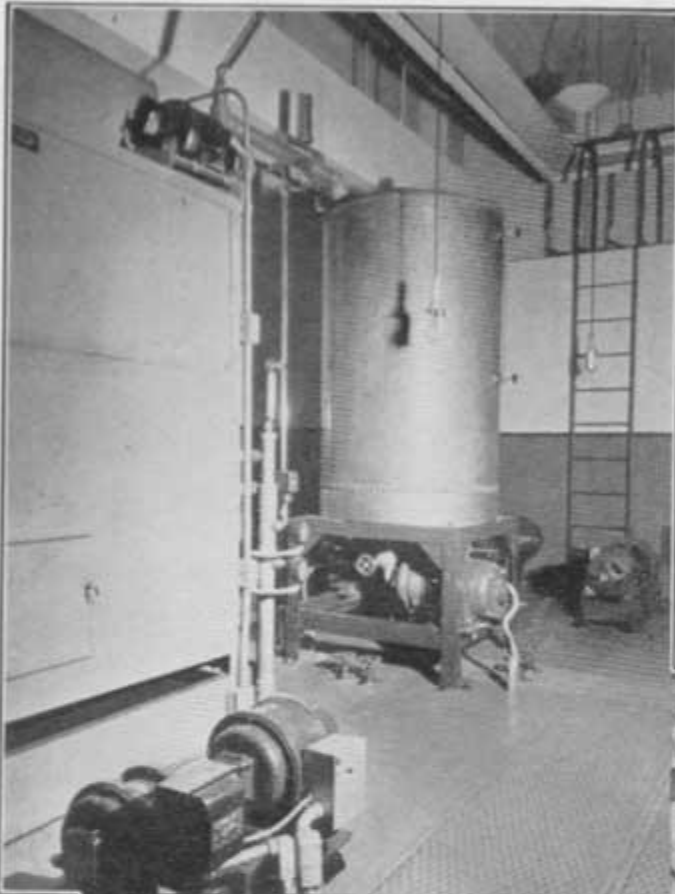
FIG. 36. ABOVE, WATER COOLING EQUIPMENT FOR THE ULTRA-FREQUENCY TRANSMITTING TUBES. THE ROUND TANK IS FOR STORAGE, WHILE THE RECTANGULAR TANK IN THE FOREGROUND CONTAINS THE COOLING UNIT.
